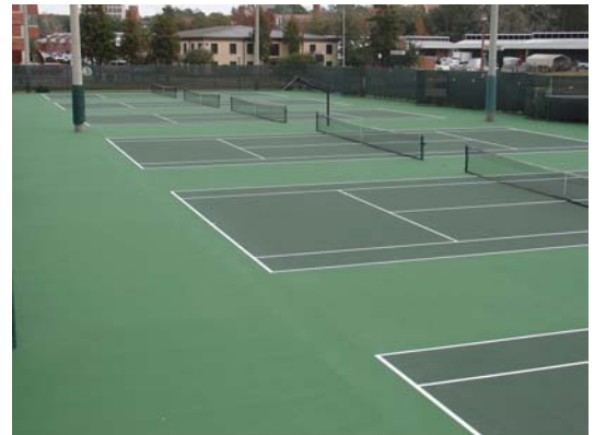
The Florida State University Tallahassee, FL Scott Speicher Tennis Center 12 asphalt courts
